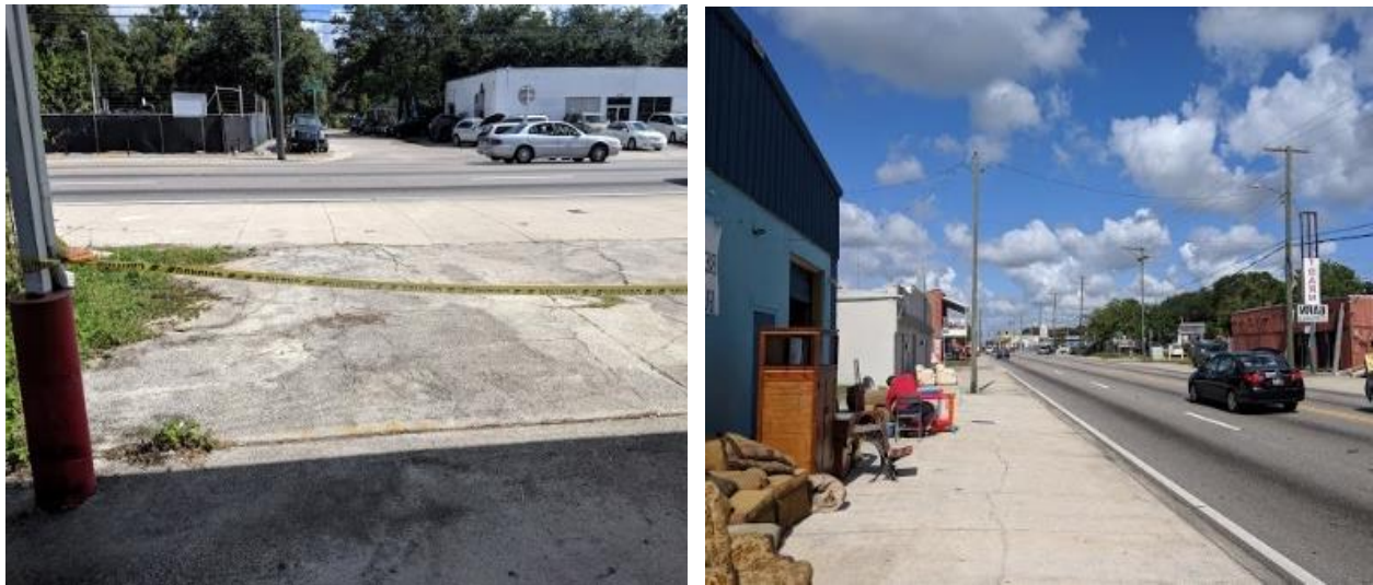
Figure 17: A closed office entrance to a mechanic shop because of flooding on Nebraska (left), and a frequently flooded furniture store on the same street (right) (Author).
