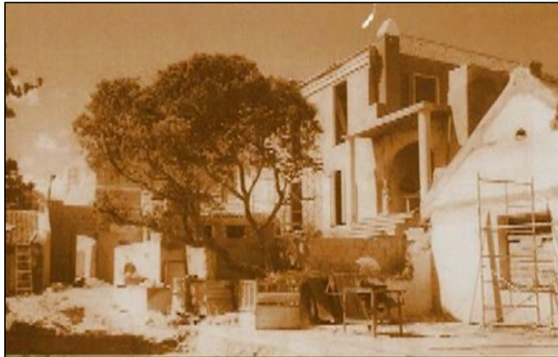
Figure 1.3. Museum Kura Hulanda reception building, entryway, and adjoining structures prior to restoration. Photo courtesy Museum Kura Hulanda.
