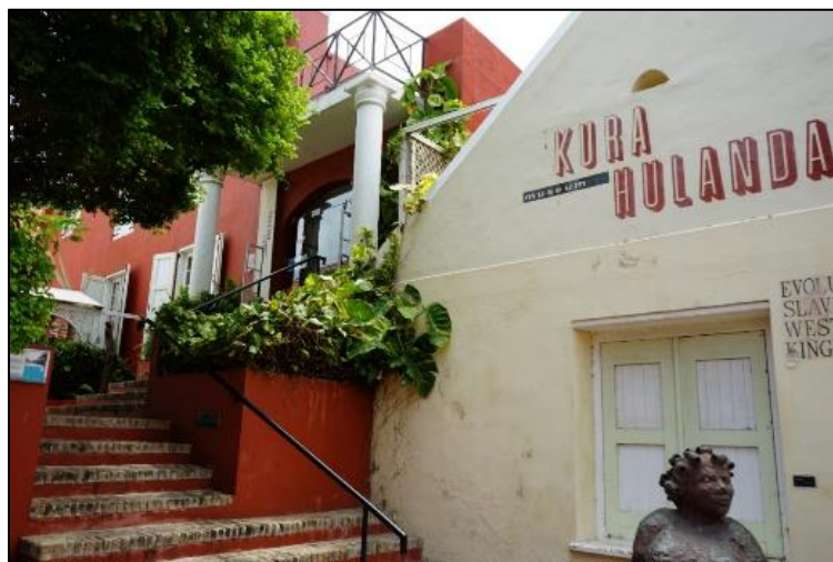
Figure 1.4. Museum Kura Hulanda reception building, entryway, and adjoining structure, July 2018, post-restoration. Photo by author.
