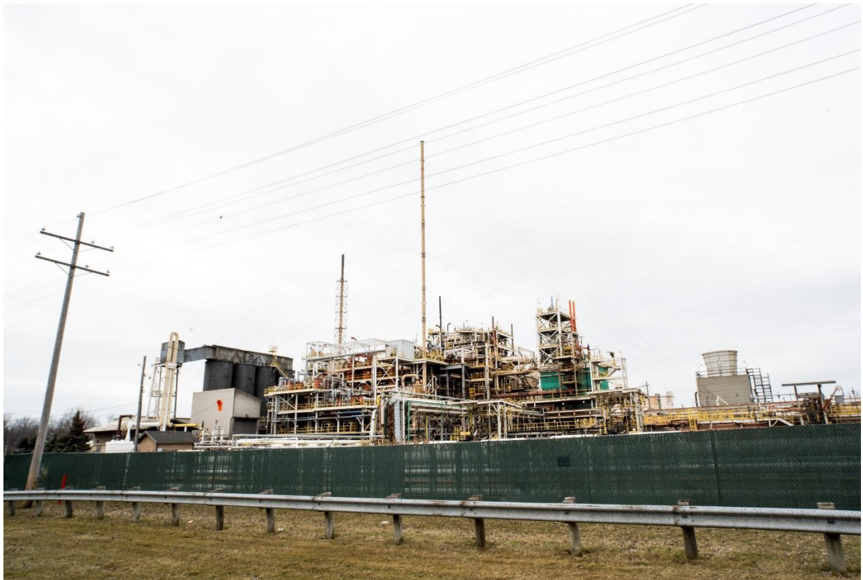
Figure 7.2: Plant 2 as seen from Middle Road. Photograph by Ryan Cook.
