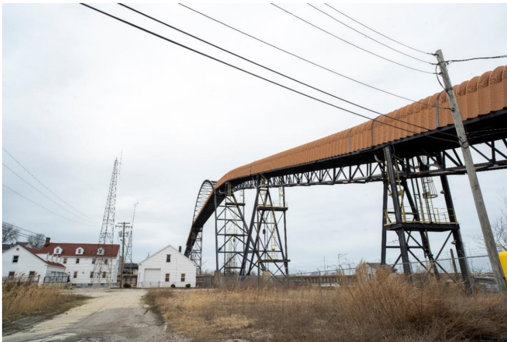
Figure 8.1: Coal chutes (seen above) were used to move coal from ships where it was delivered to railroad cars that would stack it. Photo by Ryan Cook.
