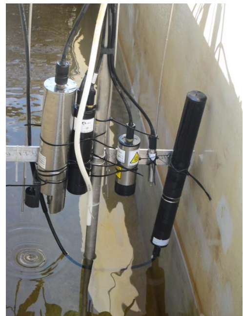
Figure 3.1. Weathered oil/dispersant mixture is poured onto the water surface on the afternoon of June 3 after wave generation has begun (above). In situ fluorometers attached to a crossbeam in the tank (right).
