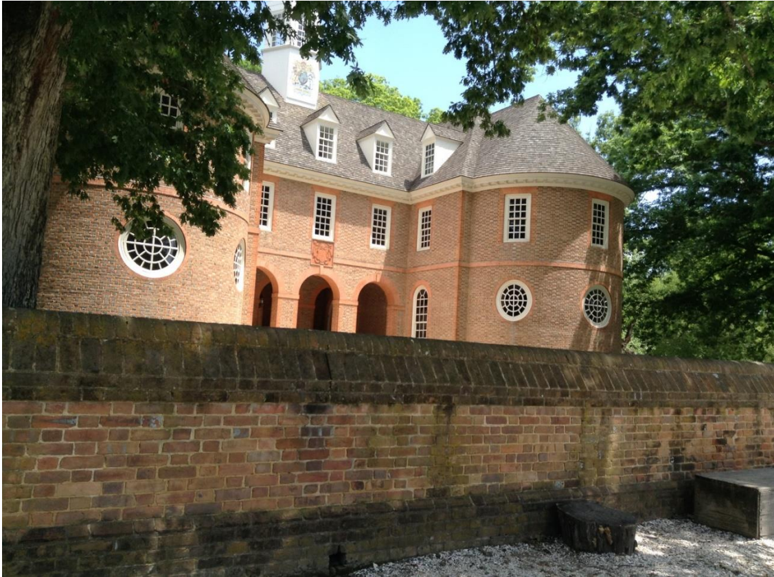
Figure 5.26. Luka’s photo entitled “America’s first Capital building.”
