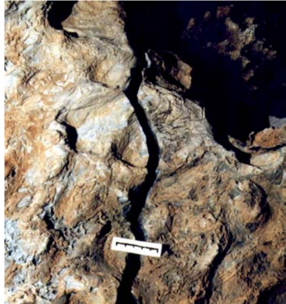
Fig. 8. Open joint at chert ceiling in Lesser Canyon, Lincoln Cave. Scale in centimetres.
