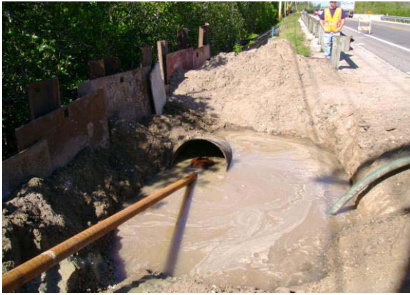
Figure 2: At the entrance the lead rod with the directional end steers the drill.
