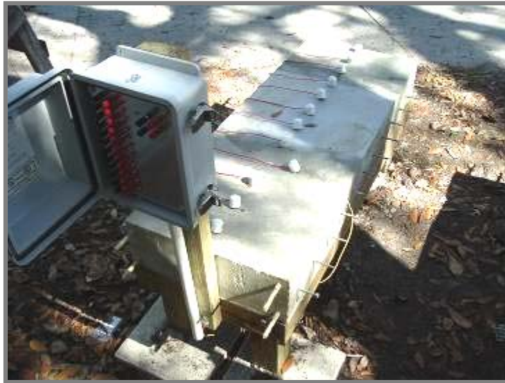
Figure 8 - Installed yard slab with connection box.
