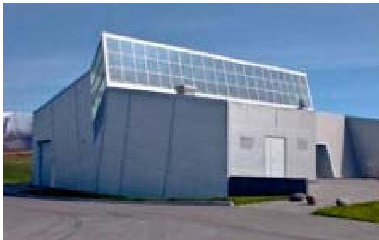
Figure 2.7 Kalina cycle geothermal power plant in Iceland [26]
