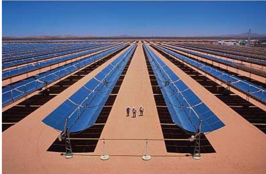
Figure 2.3 Parabolic trough solar collectors [10]
