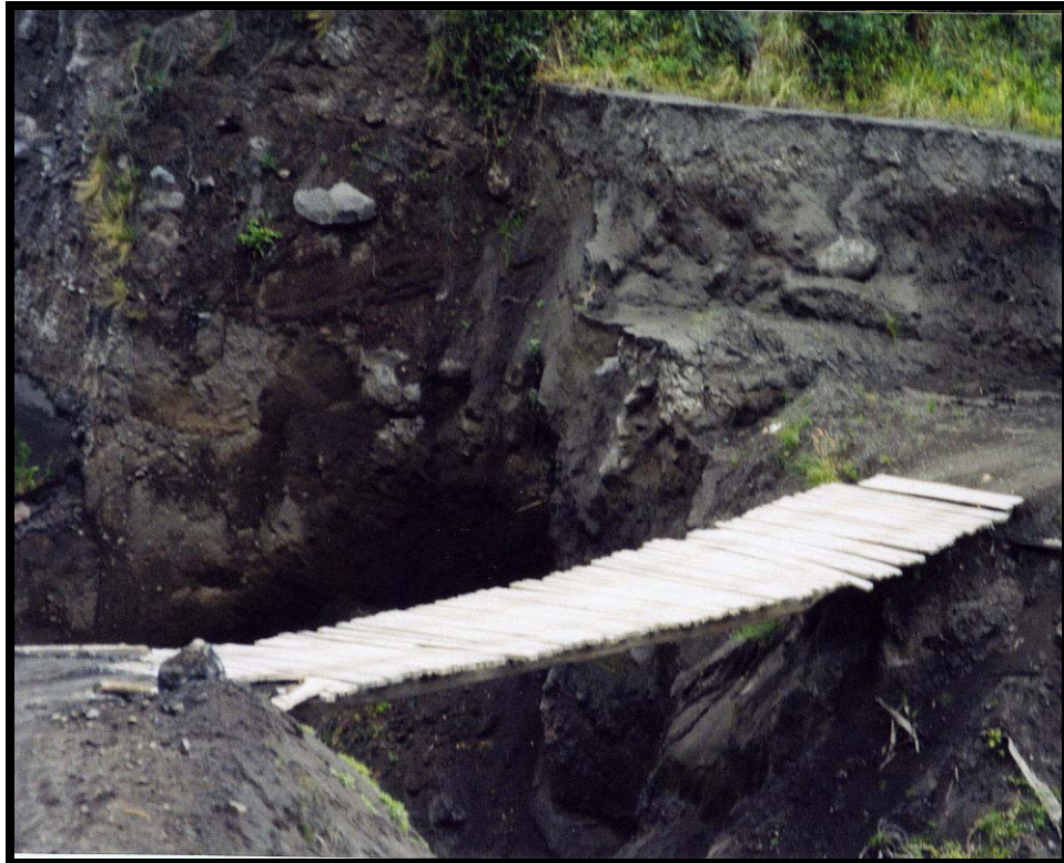
Figure 22: Bridge in Bilbao Parish
