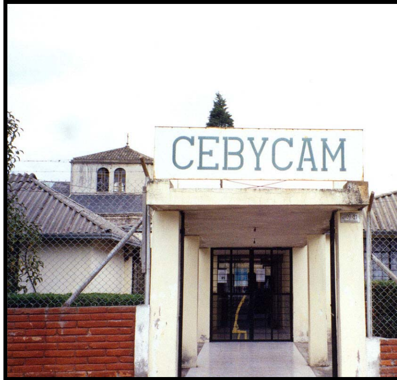
Figure 5: Entrance to CEBYCAM (monastery in rear)
