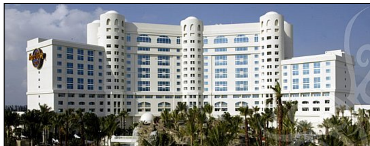
Figure 2.2: Seminole Hard Rock Hotel and Casino located in Tampa, Florida ( www.seminolehardrock.com ).
