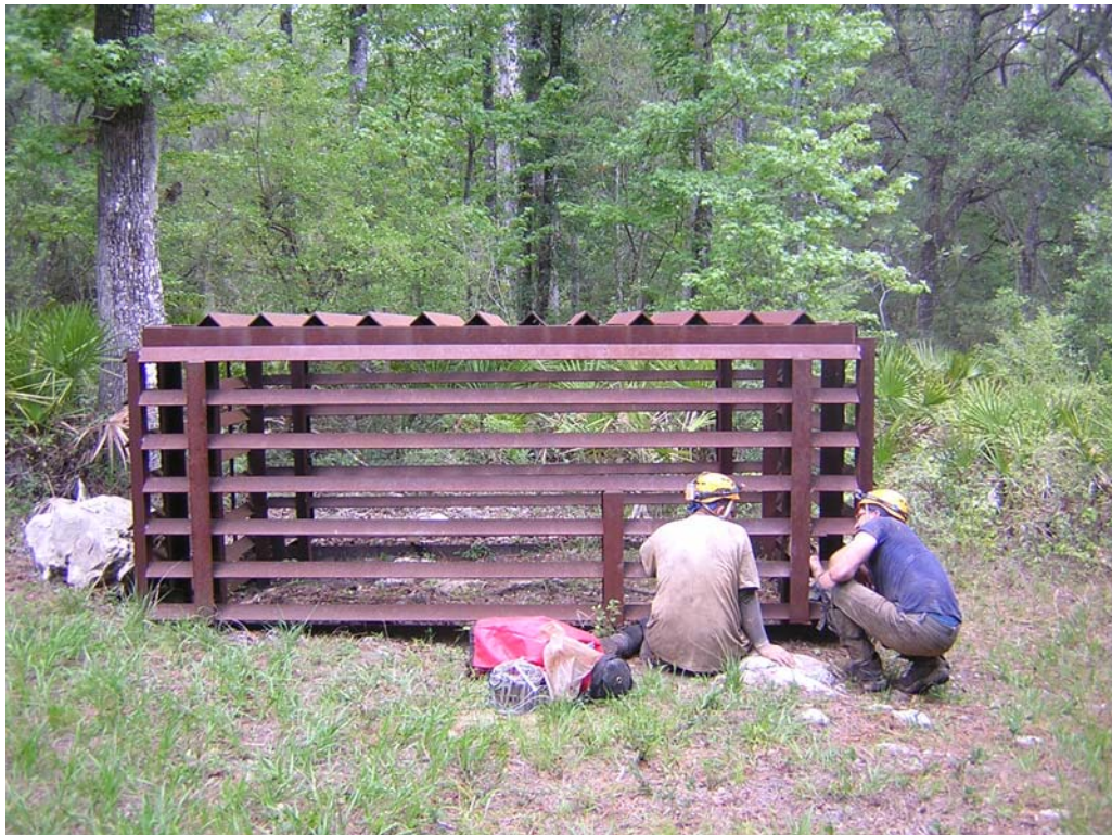
Figure 39. Blowing Hole Cave gate installed by TBAG and Withlacoochee State Forest.
