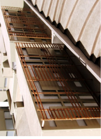
North Façade Trellises : Figure 47
