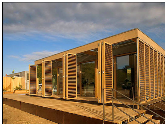
Fig.22-23 PV louver system in opened and closed positions
