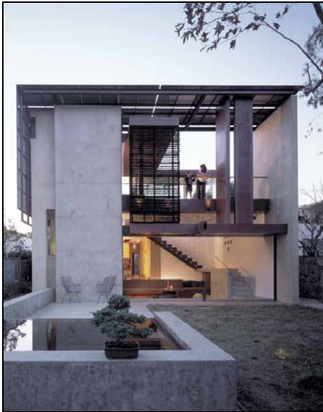
Fig.18-19 Solar arrays are located over the low slope roof area and also along the western wall.
