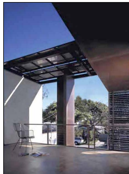
Fig.18-19 Solar arrays are located over the low slope roof area and also along the western wall.
