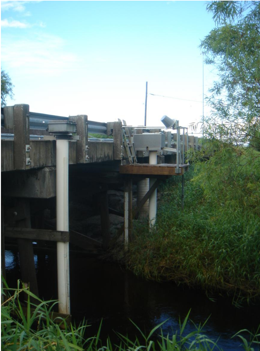
Figure 8. Picture of USGS Gaging Station. This site is number 02300700 Bullfrog Creek Near Wimauma, FL. 9/26/2009.
