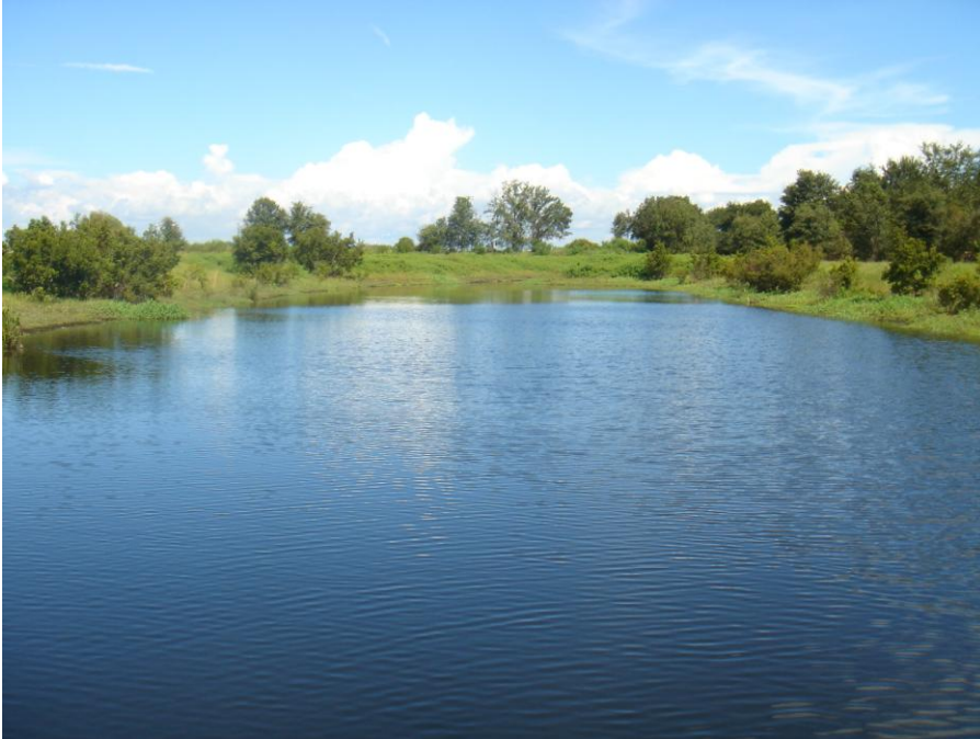
A-3. Balm Road Treatment Marsh Sedimentation Basin 9/26/2009.
