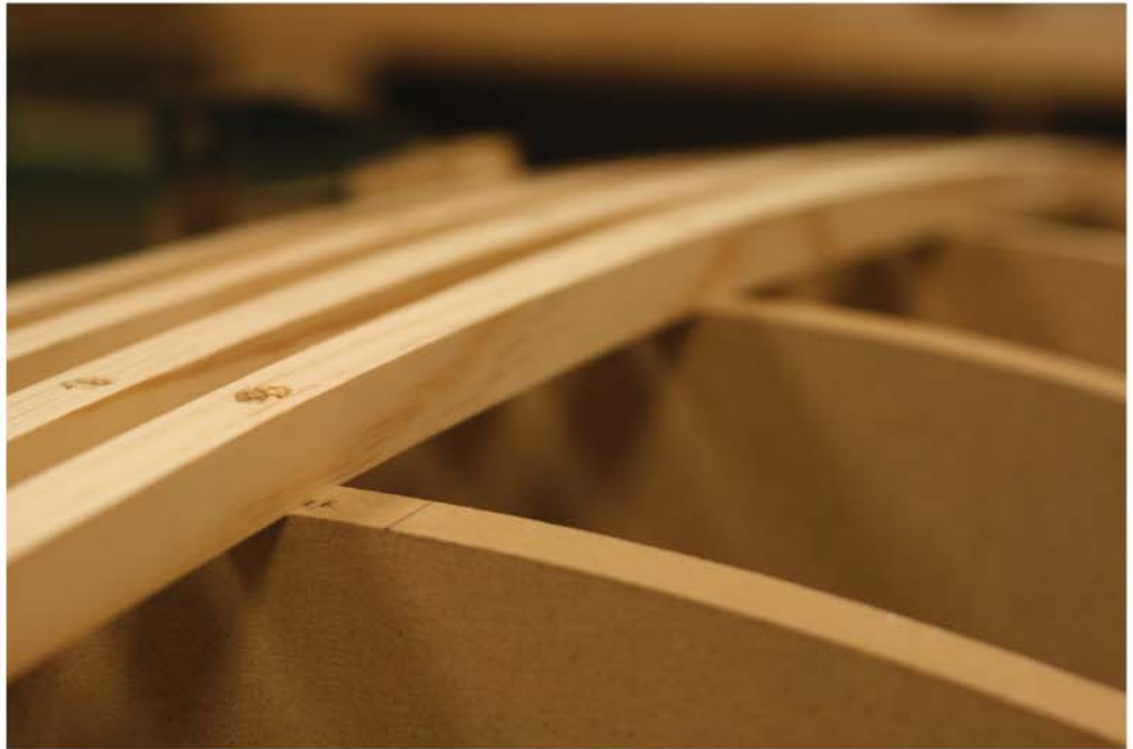
Fig. 57. Louvers sitting on compound curved columns
