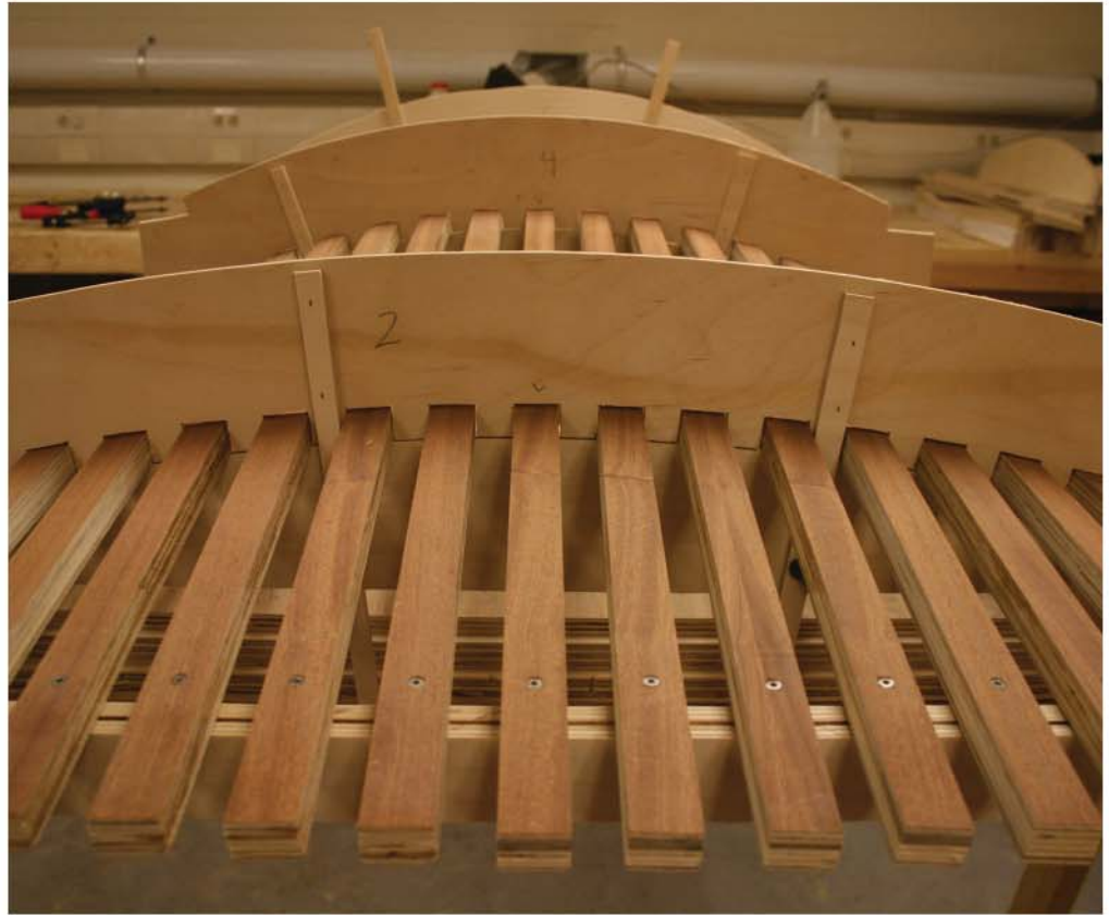
Fig. 78. Wall Assembly near completion
