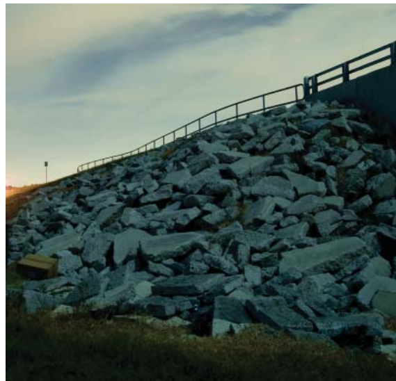
Figure 79. The hostile barriers which acts as landings for several vehicular infrastructures also acts to elevate the traveler from the grounds of his city.
