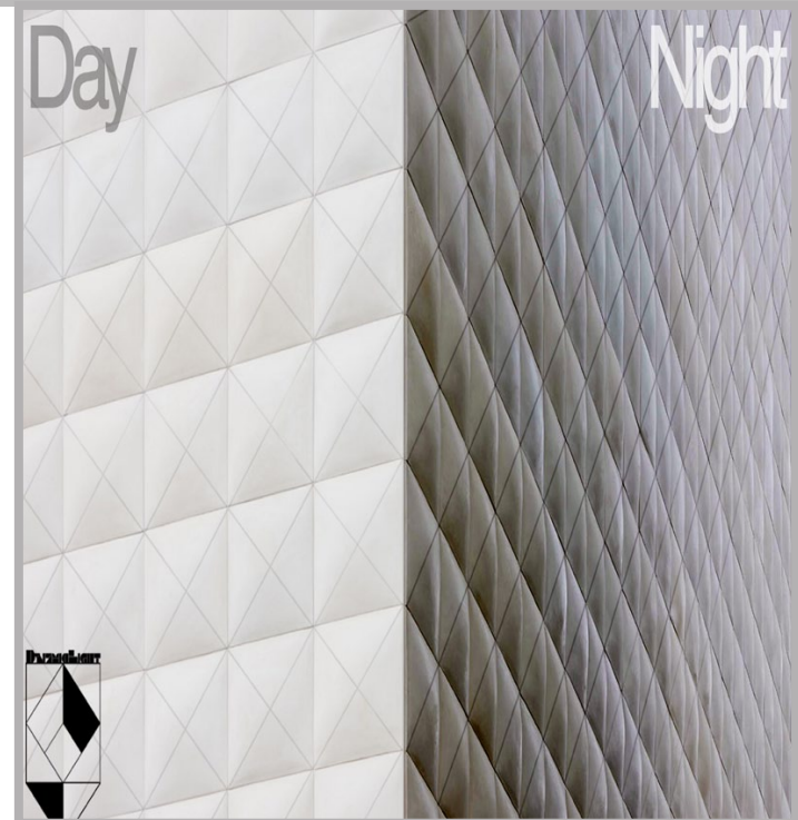
Fig.64. Day and night. The facade system has the ability to portray different things depending on its environment
