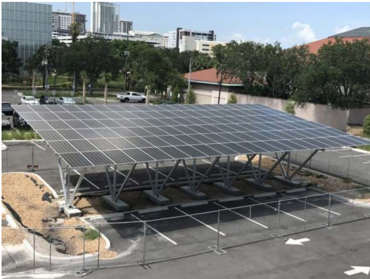
This 40kw solar array carport on campus will power 15 percent of new biology and chemistry labs. Photo by Brian Pullen.
