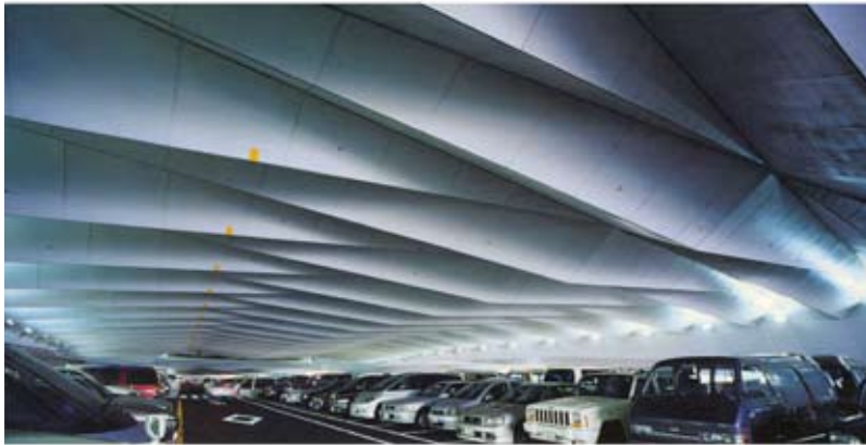
Figure 4.6. , Perspective of Garage Space With No Columns, image from Albert Ferre, The Yokohama Project (Barcelona 2002) 126.
