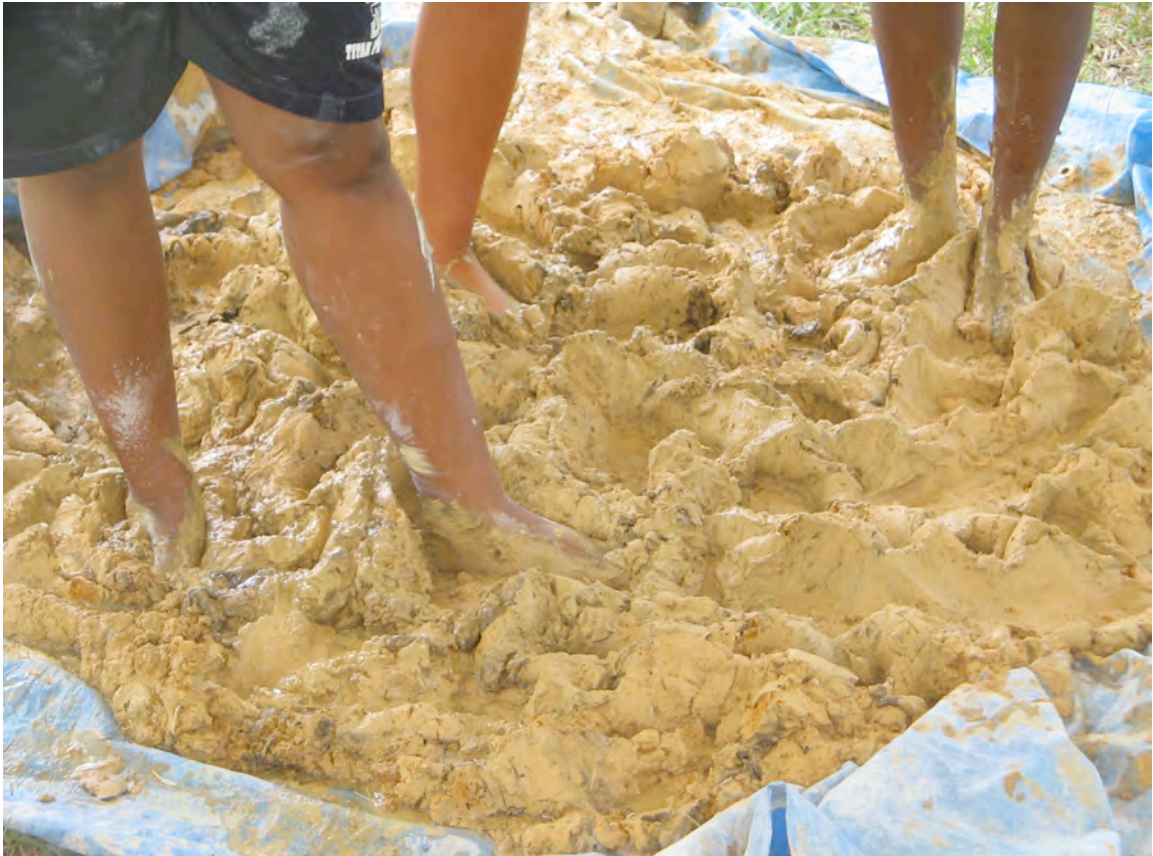
Fig. 38. On the tarp/studio: Mixing cob
