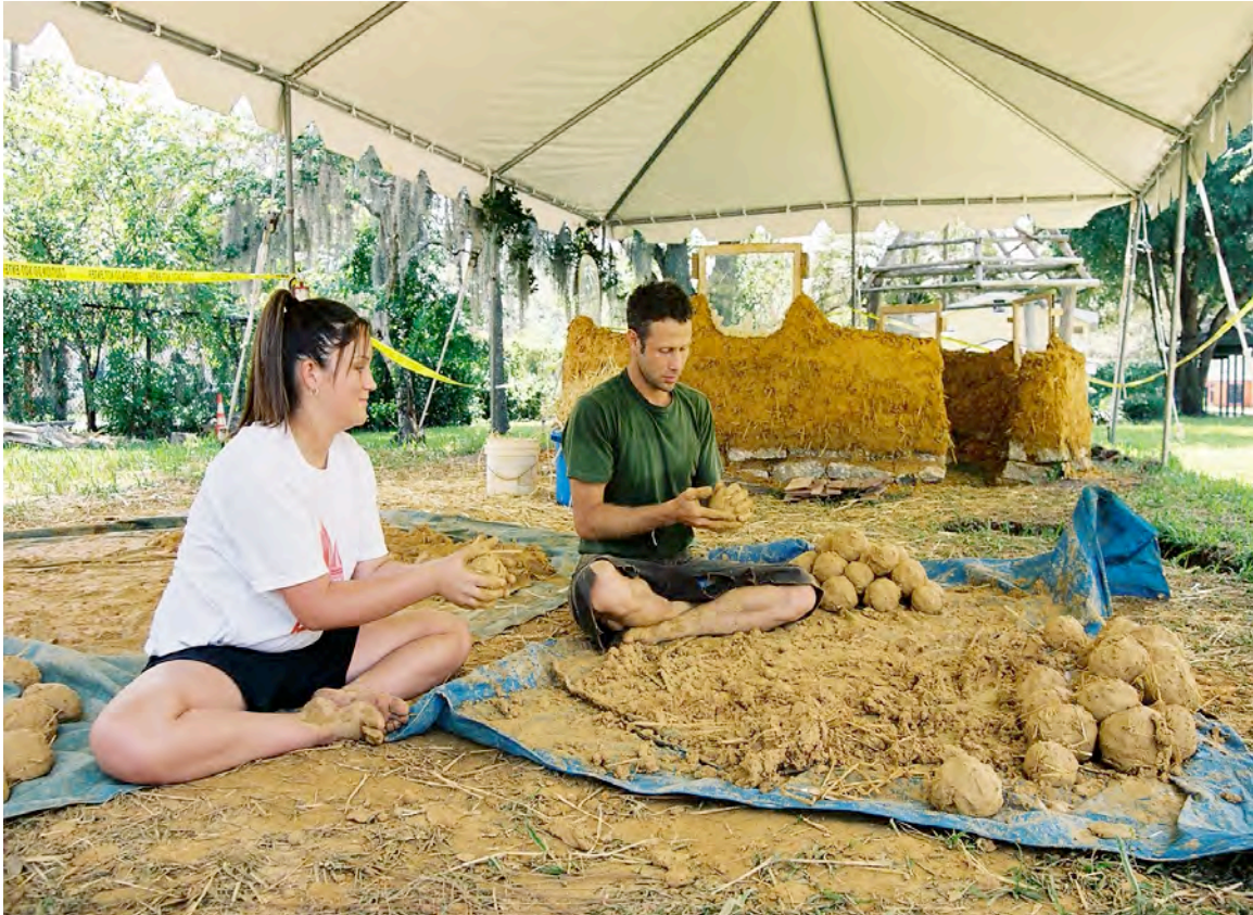
Fig. 52. Making cob balls
