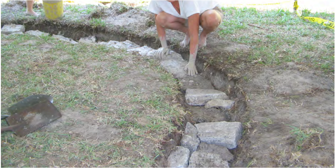
Fig. 76. Laying the shifting stone
