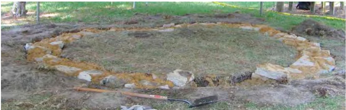
Fig. 22. Plinth wall: In the ground
