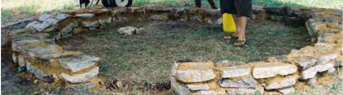
Fig. 23. Stem wall: Above ground
