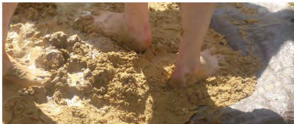
Fig. 89. Outside cobbing pile
