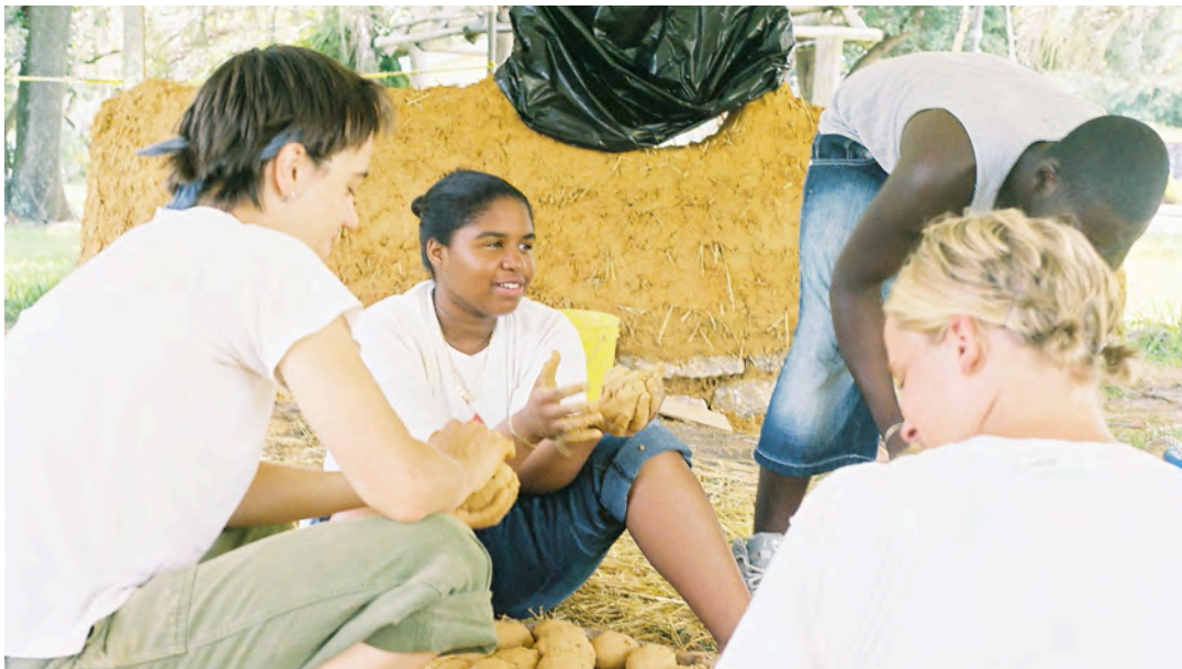
Fig. 25. Making cob balls
