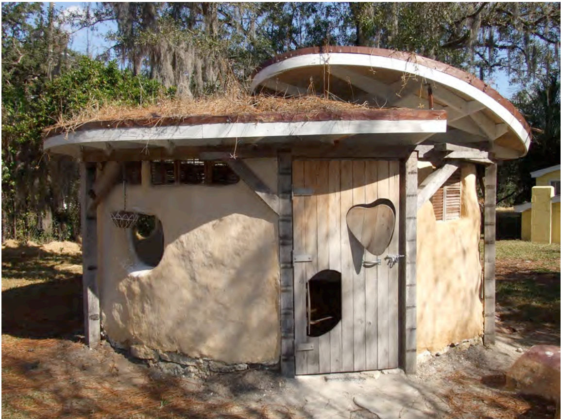
Fig. 1. Weathered cob house
