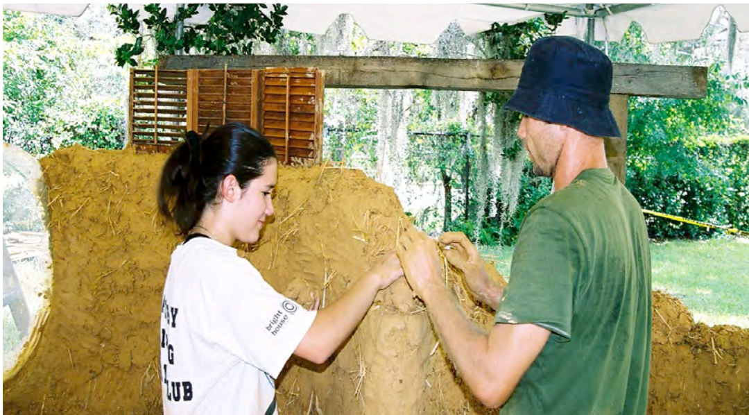
Fig. 24. Applying cob
