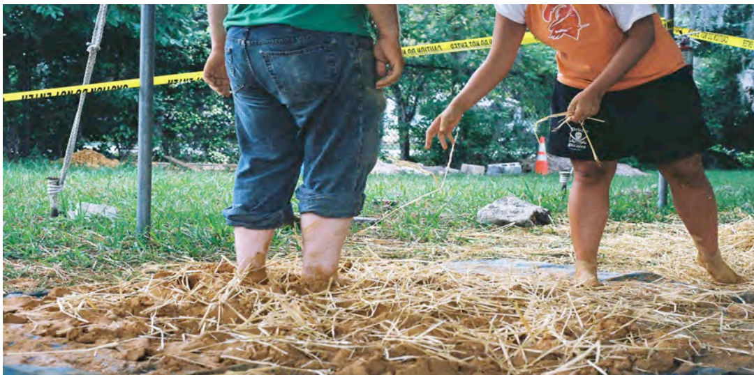
Fig. 15. One layer of straw
