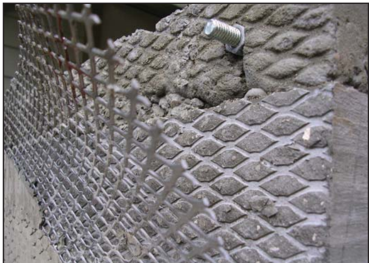
Fig. 88 Concrete showing reverse texture of screen
