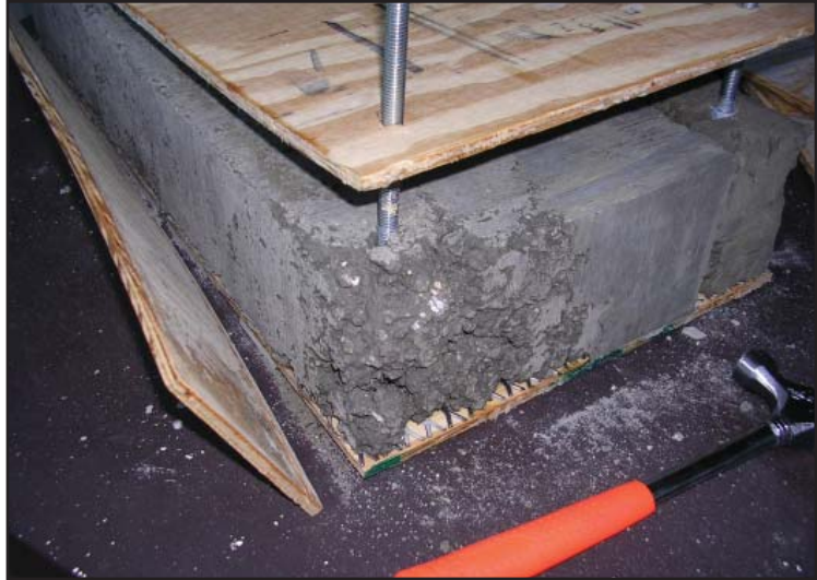
Fig. 87 Concrete sitting in the form work after our has cured
