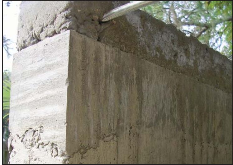
Fig. 89 Concrete showing the different pours
