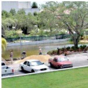
Crews work on landscaping at the University Student Center
