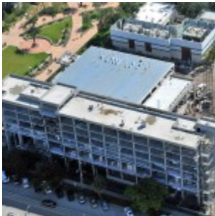
USC – November 1, 2011 | Photo: Aerial Innovations Inc
