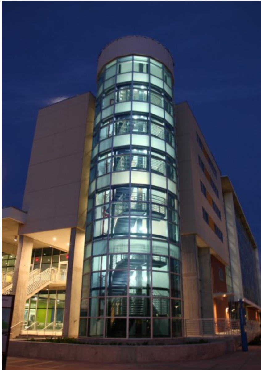
Residential tower at the University Student Center
