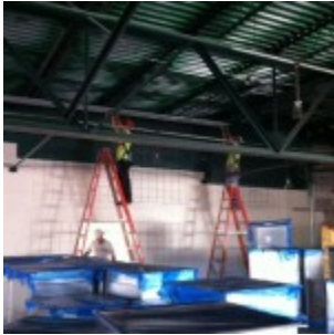
Conduit installed at Student Life Center
