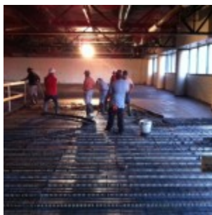
Pouring the deck at the Student Life Center
