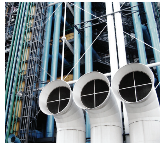
Figure 2.12. Below. Pompidou Center Detail
