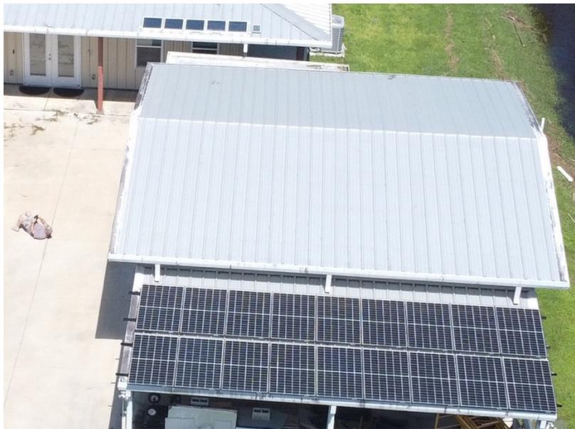
Figure 2.1 5.94 kW PV System.
