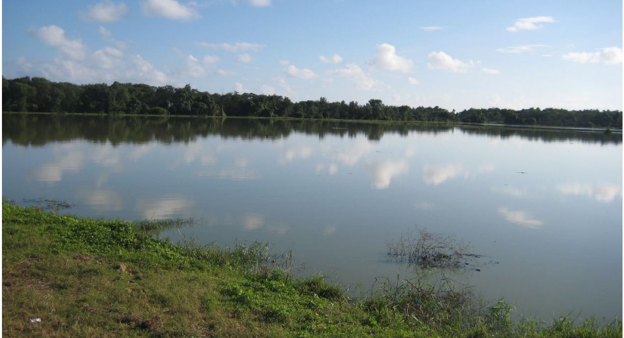
Figure 13. The main facultative lagoon at the Belize City Treatment Plant. Photo by EC Wells.
