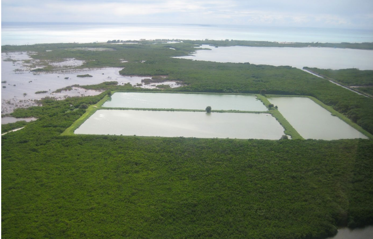
Figure 14. Facultative lagoons and maturation pond on Ambergris Caye. Photo by EC Wells
