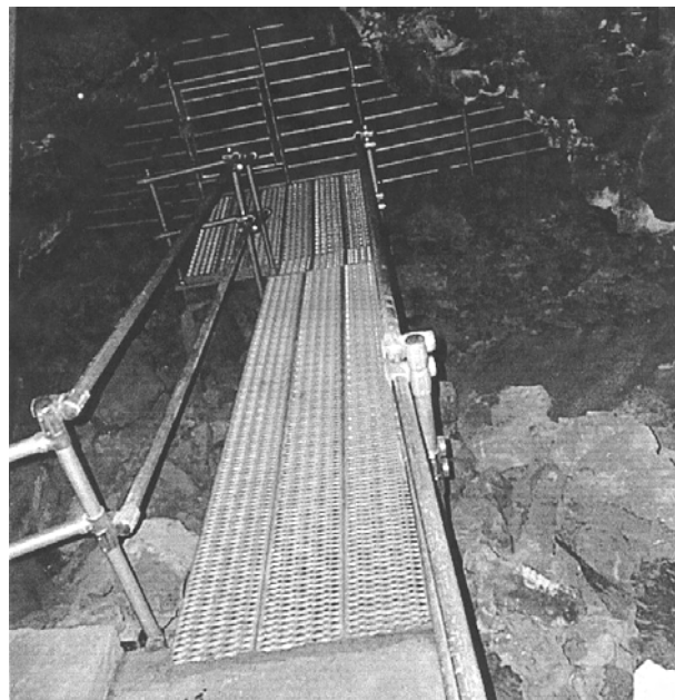
Figure 4. Viewing platform and gate in lower level of Skull Cave. The gate spans the entire passage width of four meters (14 feet) (photo by Kelly Fuhrmann).
