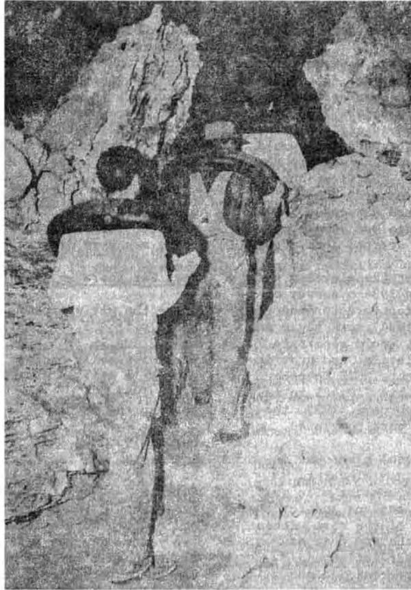
FIGURE 5. Civilian Conservation Corps workers carry concrete in tire innertubes through Wind Cave to where another step will be poured. (Photo courtesy National Park Service)
