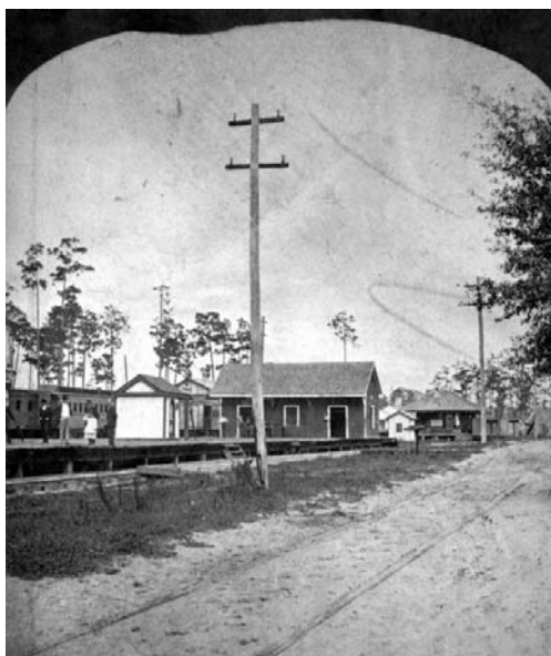
figure 15. Live Oak Rail Station 1877 79
