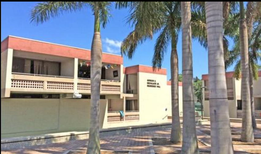
Figure 28. New College (Photo Courtesy of David Pierson).
