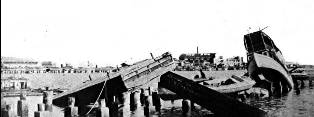
Figure 35. Municipal Pier Damaged by 1921 Hurricane (Courtesy of St. Petersburg Museum of History).
