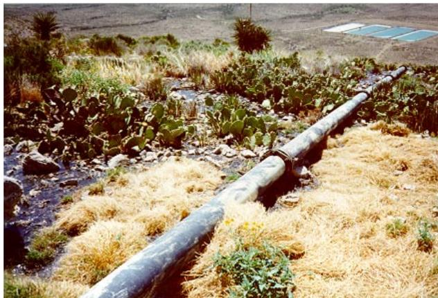
Main sewer line leak discovered in early June, 1998. Sewage is flowing from left of photo. Note sewage lagoons in the background. (NPS Photo by Dale Pate)
