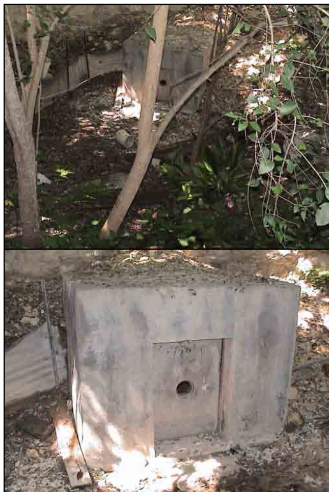
The Robber Baron Cave Entrance: sinkhole (top) and bunker closeup (bottom).
