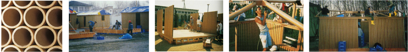
Figure 28. Construction of paper log houses.
