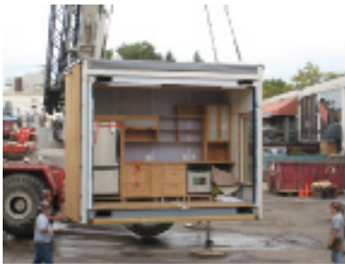
Figure 44. Construction of triPOD prefabricated modular system.
