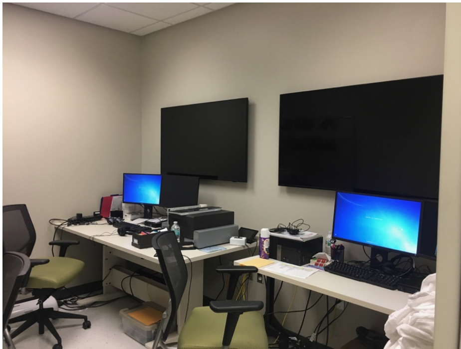
Figure 3.2 The Video Monitor Room
