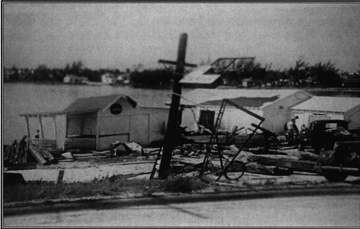
Steve Lowe's home and his father's fish house, located on the mainland (west side) of the old South Bridge in Fort Pierce, were damaged in the hurricane of 1949.
