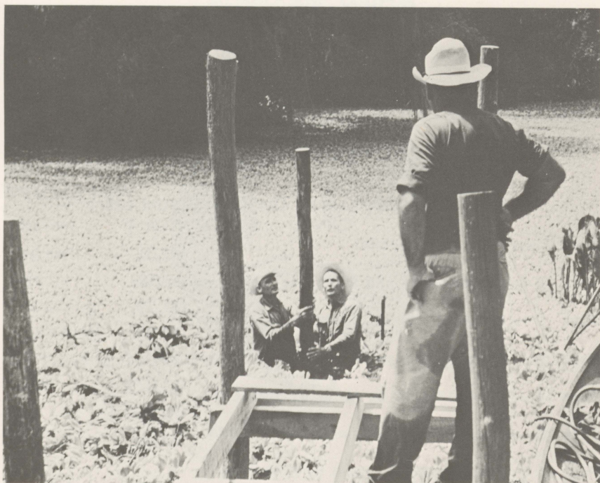
Building the Boardwalk
