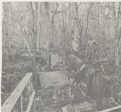
Hurricane Damage (Donna)
