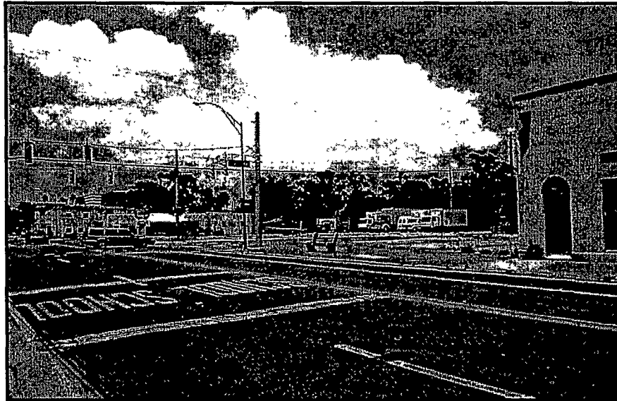
Figure 51. Existing conditions on South Fort Harrison Avenue
