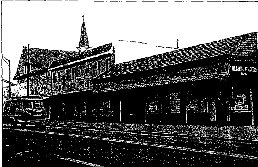
Figure 11. Underutilized retail opportunity on South Fort Harrison Ave.
