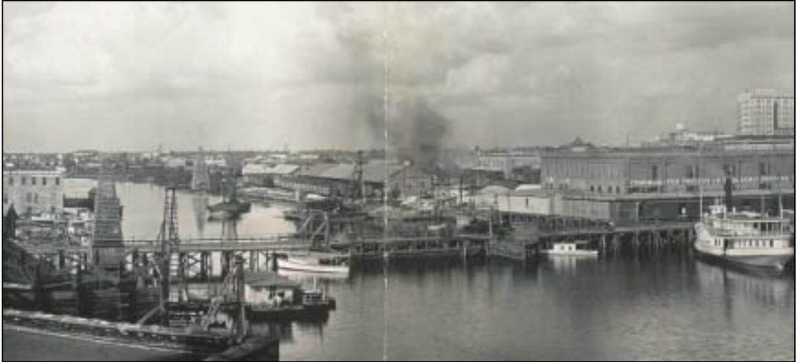
**Figure 10.** Detail from a February 1913 photograph of the temporary bridge crossing the Hillsborough River at Jackson Street. The Lafayette Street Bridge has been demolished, and equipment barges and piles of construction materials can be seen in the center of the image where the east approach is under construction
