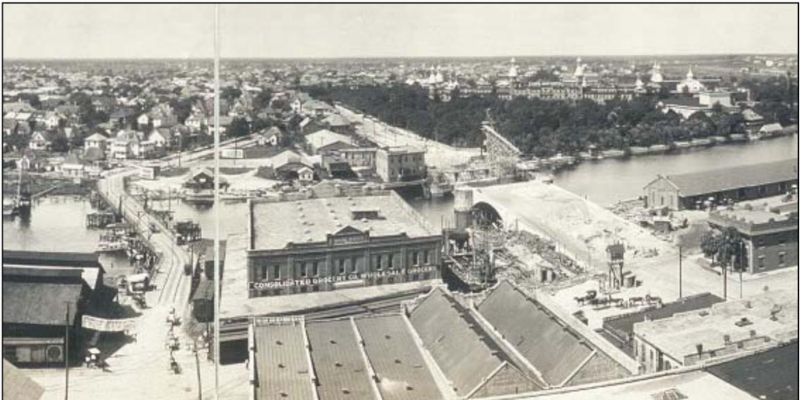
**Figure 11.** Detail from an October 1913 photograph taken facing west from the Mudge Building in downtown Tampa. The temporary Jackson Street Bridge is to the left, and the Lafayette Street Bridge is to the right. The concrete for the east approach and the east arch has been poured, and concrete work is progressing on the west side of the river
