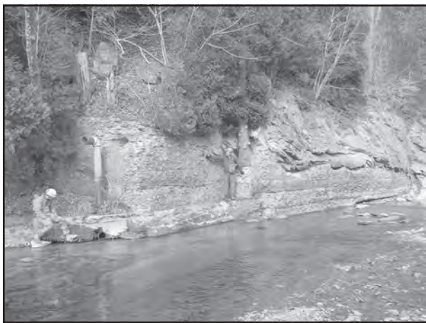
Figure 1: A stream issuing from a cave was formally used as a town's water supply. To create a reservoir a concrete dam was constructed across the cave entrance to impound the stream. The cave stream now flows beneath the abandoned dam.
