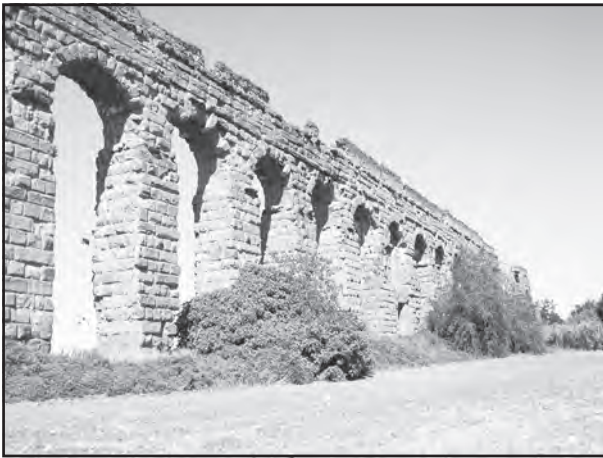
Figure 1: Above ground arcade section of an aqueduct near Rome (photo: C. Galeazzi).
