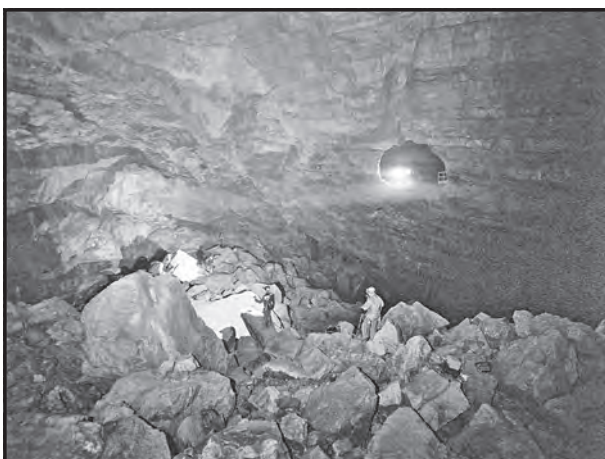
Figure 2: Cave chamber in highway tunnel.
