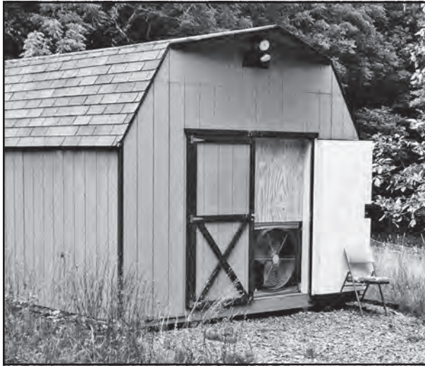
Figure 4: Inside this shed used for apple storage is Big Bucks Pit, a 43 m. drop into Barberry Cave. The pit is sealed to the floor of the building. The door to the building has been reduced to the size of the fan. Accordingly, as the fan blows in and out of the building the air is exchanged in the cave.
