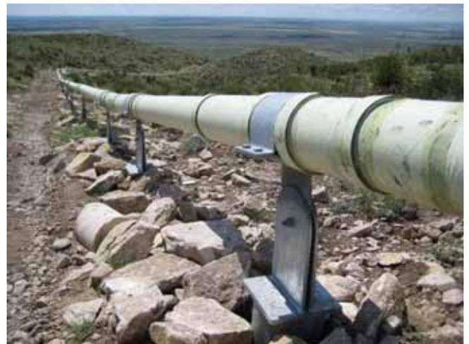
*The new above ground sewer line installed so it is not on top of the Left Hand Tunnel and Bat Cave in Carlsbad Cavern. Photo by Stan Allison.*
