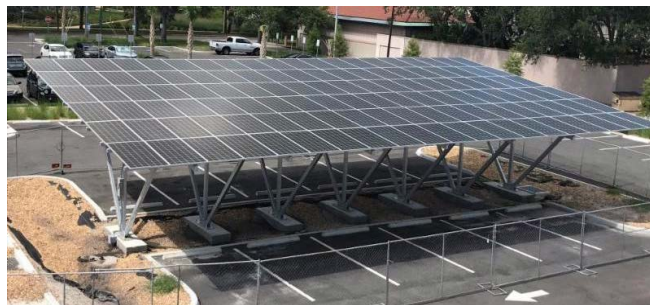
This 40kw solar array carport on campus will power 15 percent of the new Poynter Warehouse Labs. Photo by Brian Pullen.
