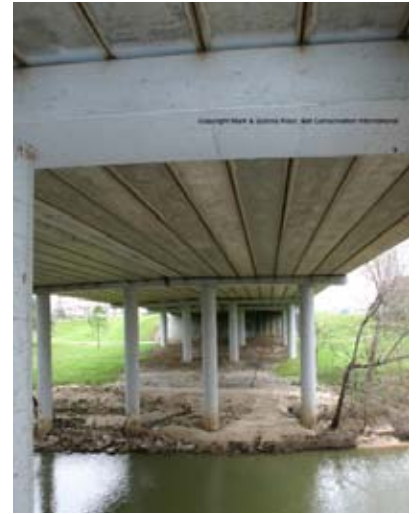
Waugh Street Bridge.
